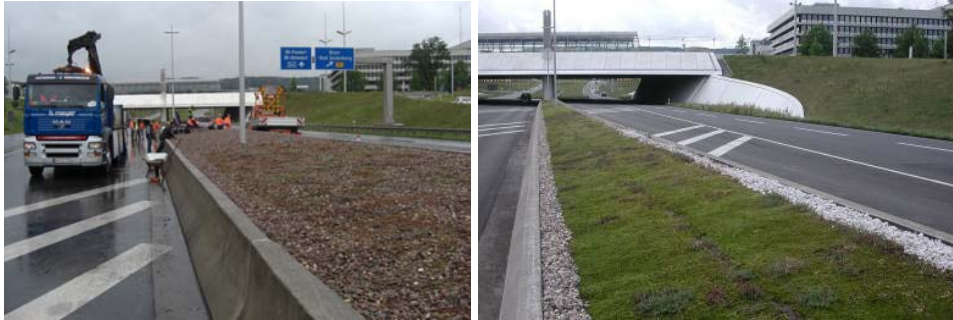
Enka ® -Moss after installation at A562 near Bonn (D)
